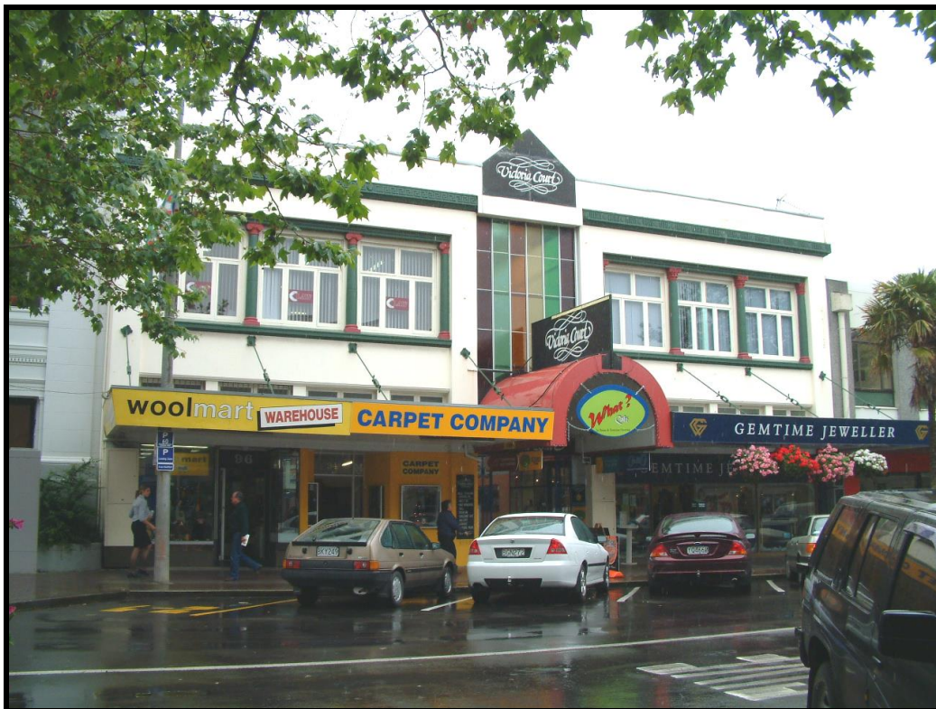
Victoria Court, the right side built for the Wanganui Meat Freezing Co and the left formerly the offices of Norwich Union Insurance (B17 18n).
