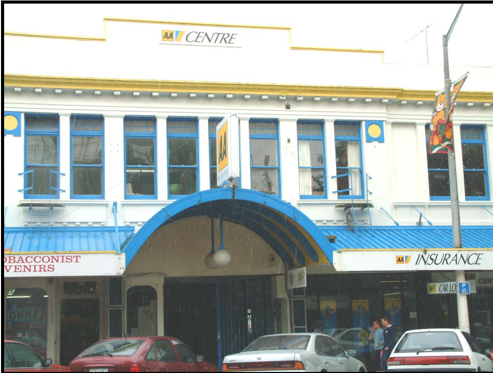
Verandah altered for AA Centre entrance (B17 16n03).
