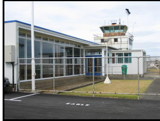
The terminal and control tower viewed from air-side. Note the atrium for passengers, an addition to the original building, which once had a viewing platform on the roof.
