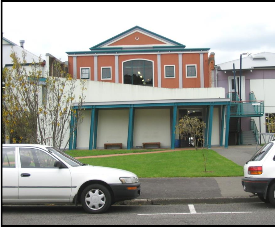
The rear view of the rebuilt Cock & Co building.
