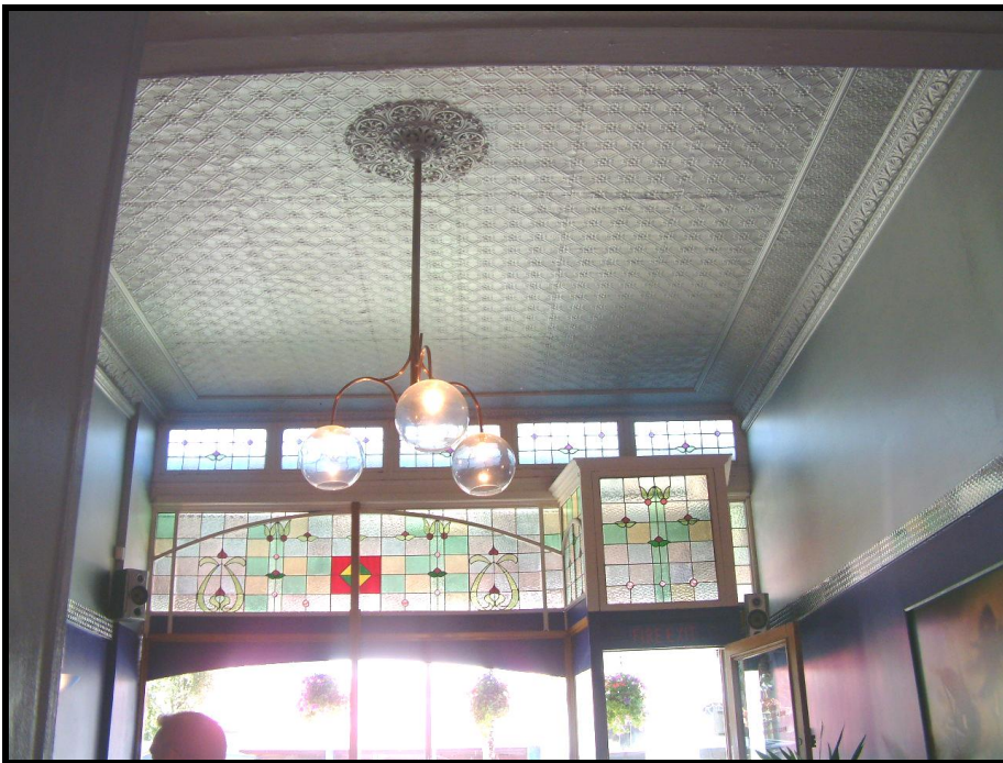
The pressed tin ceiling and Hughes Allomes & Tarrant stained glass leadlights in Drew’s (B6 7o).
