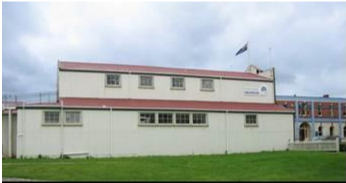
A side view of the original part of the Rowing Club building
