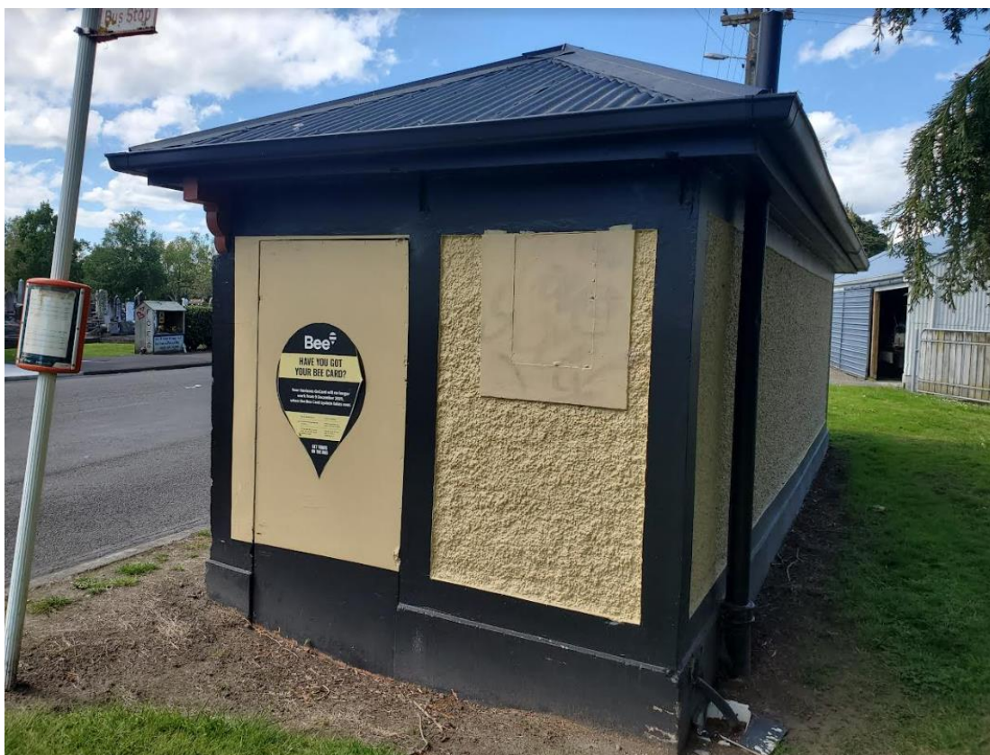
Fig. 3: At the south end of the terminus shelter at 462 Somme Parade by the Aramoho Cemetery, (historically referred to as the Aramoho Park Shelter), the boarded up public toilet remains in situ. It's unknown when this was closed off to the public.
