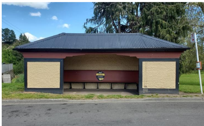
Fig. 1: The terminus shelter at 462 Somme Parade by the Aramoho Cemetery, historically referred to as the Aramoho Park Shelter. Photographed 4.10.2024 by Scott Flutey.
