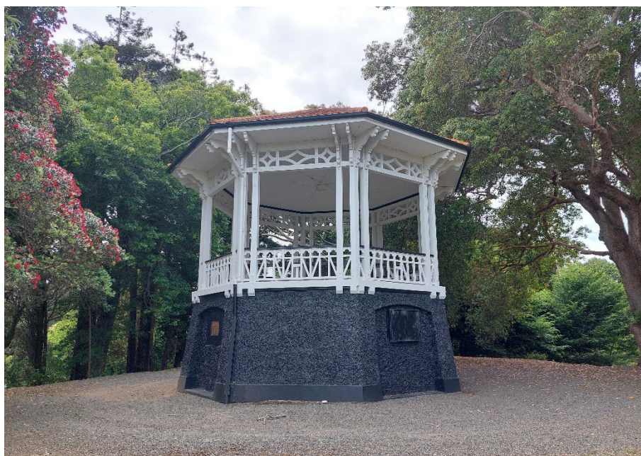
Fig. 2. Looking roughly east towards the western elevation of the Coronation Band Rotunda at Rotokawau Virginia Lake (December 2023).
