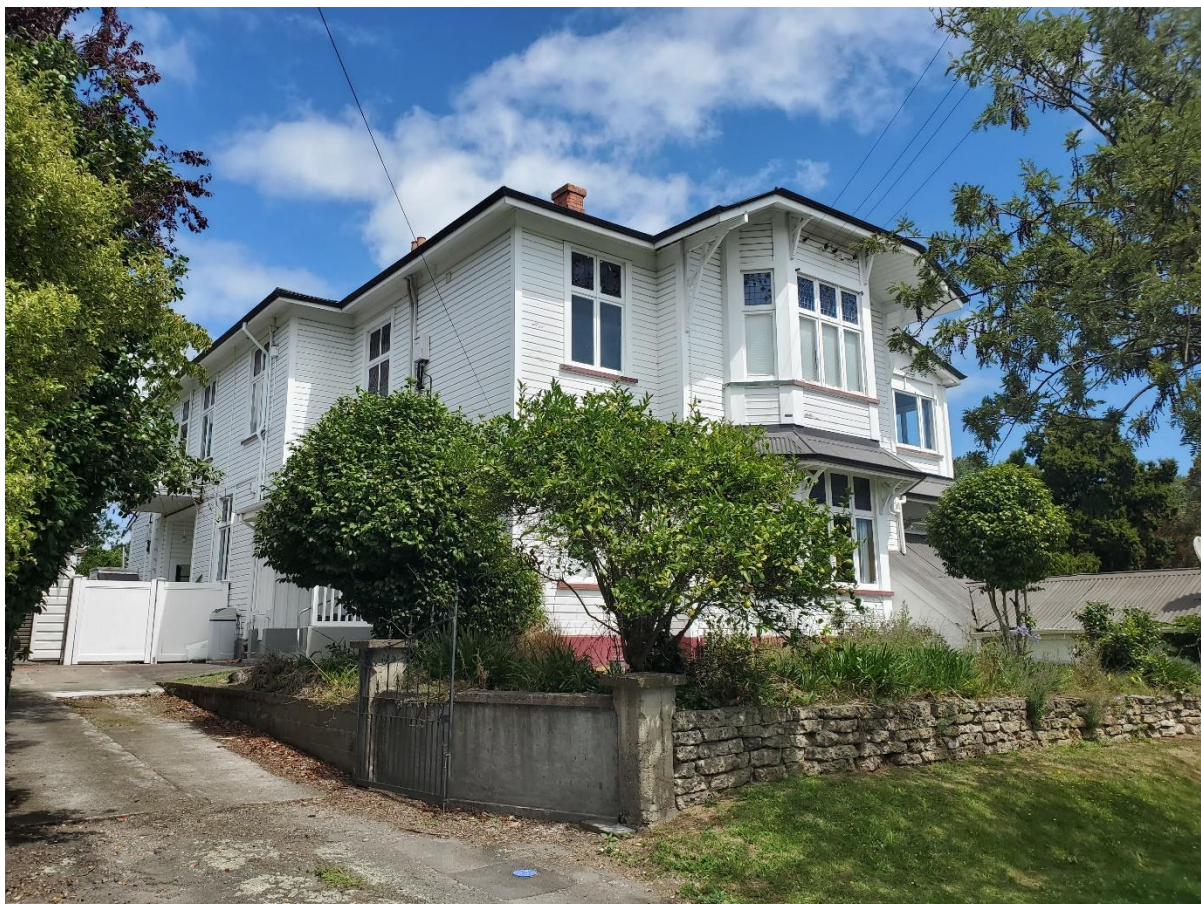
North-facing elevation of the house including the rear entrance with rendered fencing allowing drive-on access. Leaded fanlights are placed over each side-opening casement window – this is an uncommon level of ornament helping to elevate the homestead above more typical suburban villas and early bungalows built in the years leading up to the First World War. Photo taken 31.1.2024.
