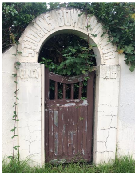
Entrance gate to the bowling club, 6 April 2022.
